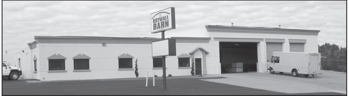
The Drywall Barn renovated this building at 408 North Meridian Road for its new location.
